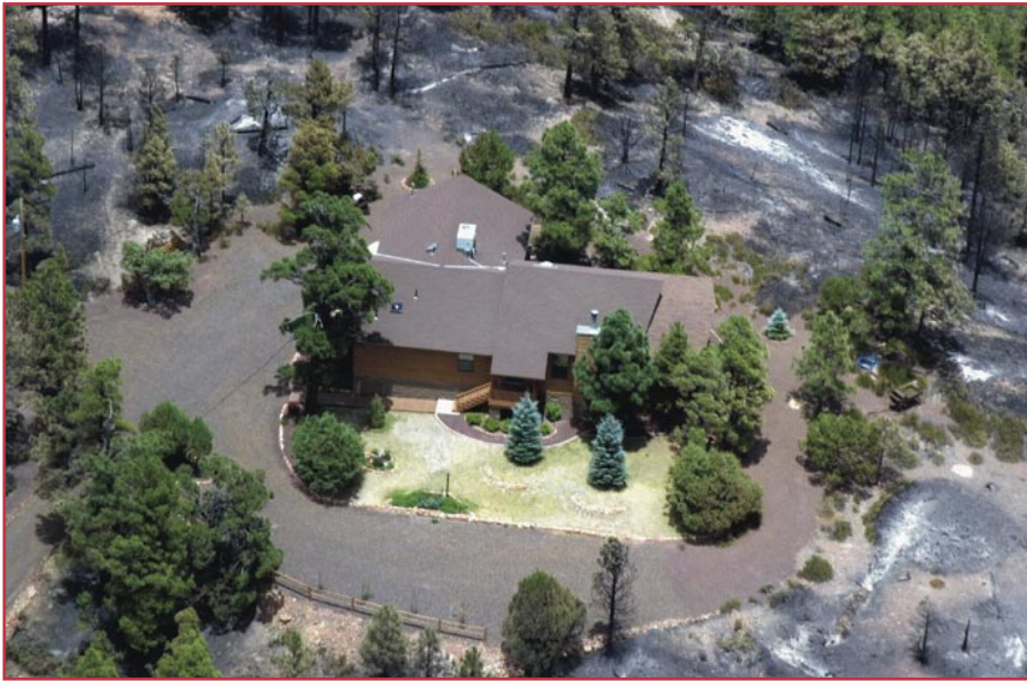
Figure 2—The Rodeo–Chediski Fire burned around this house but left it untouched, despite adjacent ornamental trees. The wide circular defensive space, coupled with adjacent cleared, open spaces, probably saved the home. Photo: Tom Iraci, USDA Forest Service, Pacific Northwest Region, Portland, OR, 2002.
