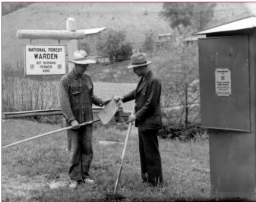
A Forest Service fire warden (left) examines a flapper, a tool used to fight grass fires, on the Hoosier National Forest in 1937. The man with him holds a broom rake, used for leaf fires. On the right is a fire cache, a tall red metal bin. Each fire cache held enough tools and water for a 10-man fire crew. Photo: USDA Forest Service, 1937.
