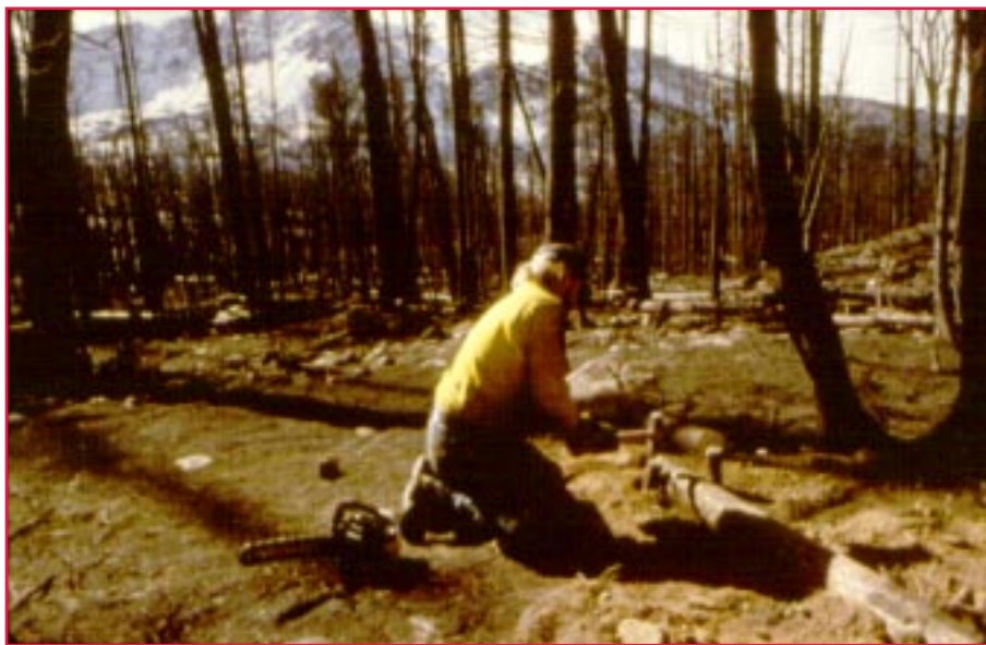
Using felled timber to control soil erosion following the 1988 Yellowstone Fires on the Gallatin National Forest, MT. Burned Area Emergency Rehabilitation teams continue to use similar techniques to rehabilitate burn sites nationwide. Photo: Ron Nichols, USDA Forest Service, 1988.
