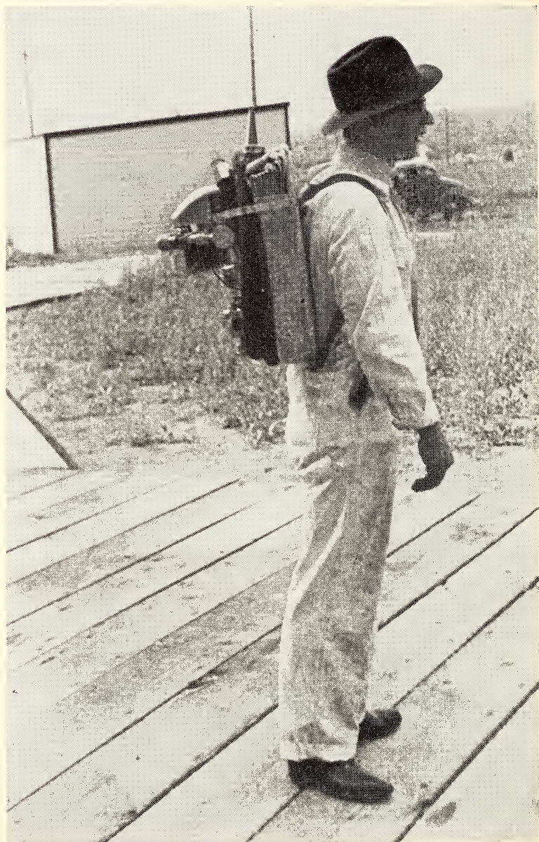
Portable pump and hose as carried on back.
