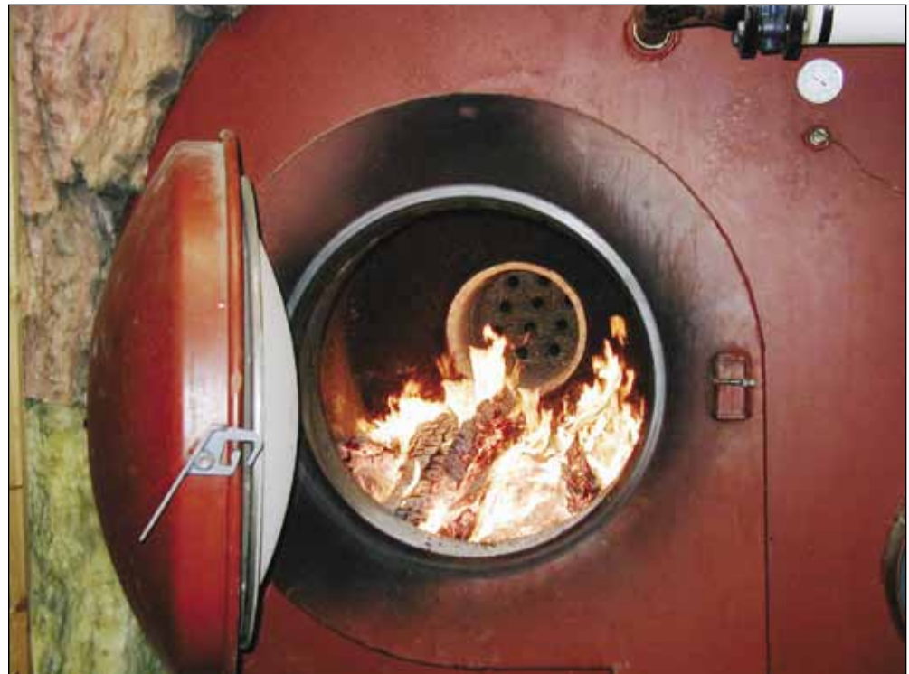
Figure 5—High-efficiency cordwood burner in Dot Lake, Alaska. The combustion chamber is surrounded by a water reservoir, which stores heat generated from the burning cordwood.
