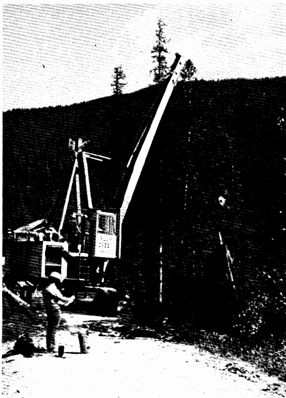
Figure 1.--A running skyline system was employed on the Coram site to provide both up- and downhill yarding capability.
