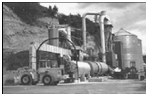
Figure 22. A Front-End Loader, Rotary Dryer, and Metal Silo Storage System.
