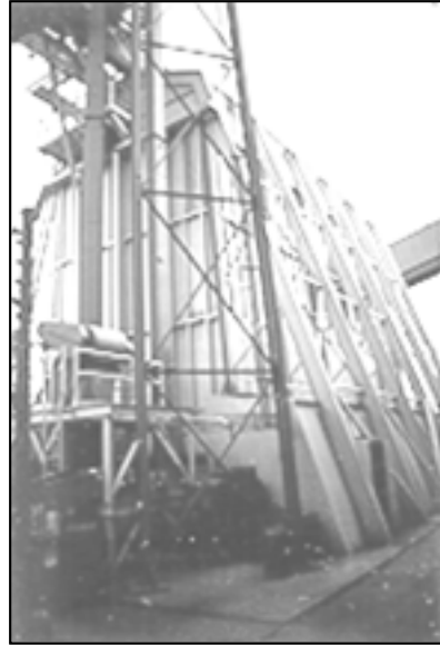
Figure 15. An Enclosed Metal Bin with a Traversing Auger Unloader.
