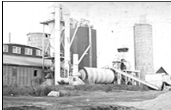
Figure 23. A Rotary Drum Drying System Showing Ducting and Particulate Capture System.
