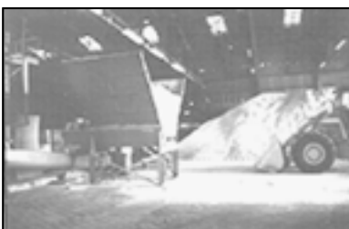
Figure 26. A Front-End Loader, Storage Pile in Building, and Feed Hopper with Live Bottom.
