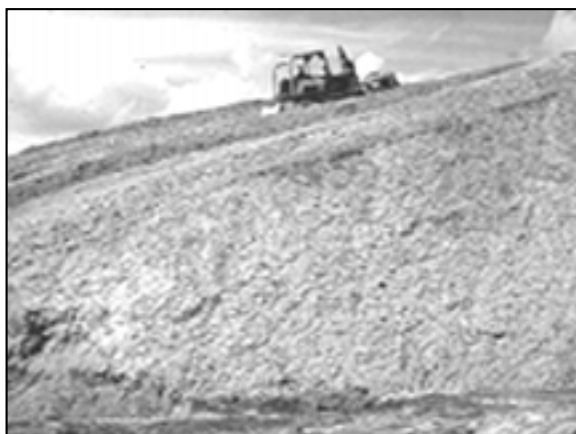
Figure 20. A Very Large Open-Pile with Bulldozer Managing the Pile.
