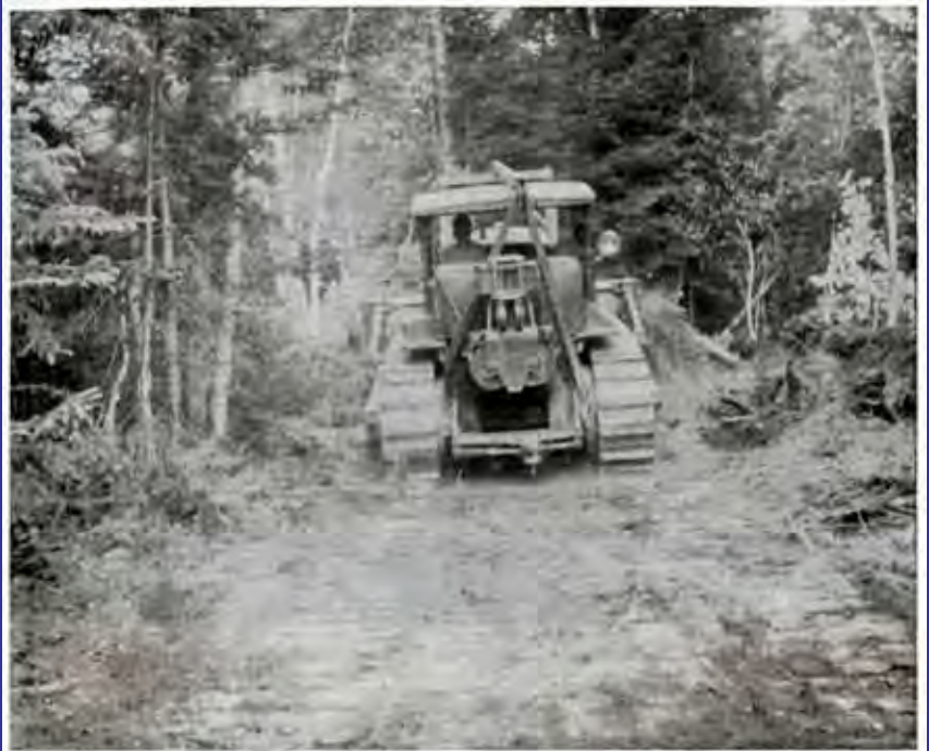
Tractor with Bulldozer building fire trail around a forest fire. Trucks with tanks of water and pumps are brought in along the trail to prevent the fire from crossing the trail and to extinguish it.
