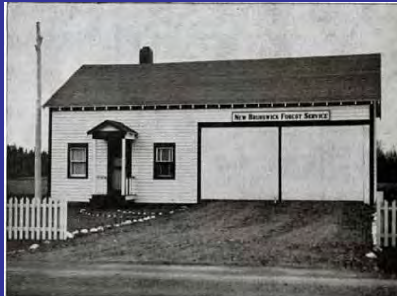
This type of building is most satisfactory for Ranger Headquarters and Equipment Depot.
