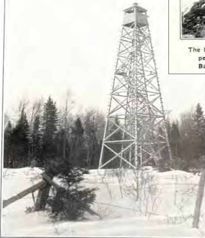
80 foot look-out tower on Ashton Hill, Northumberland County. A similar tower 90 feet high has just been completed about 6 miles east of Red Pine in Gloucester County, and a 60 foot tower on Quisibis Mountain, Madawaska County. Extensive areas are visible from all these lookouts
