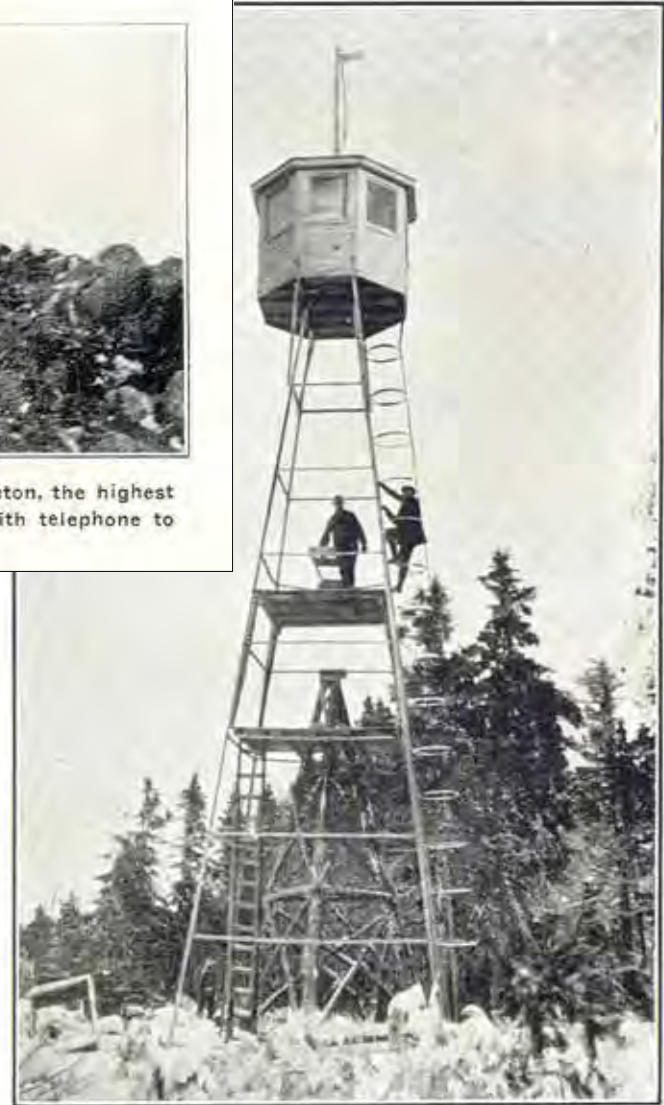
Steel Tower erected on Blue Mountain in 1923. Blue Mountain is situated at the head of the Benjamin River in Restigouche County. Elevation 1800 feet. Twelve miles of woods telephone line was built. The Geodetic Survey co-operated in the erection of the Tower and the Louison Lumber Company in the free use of their five mile private telephone line.
