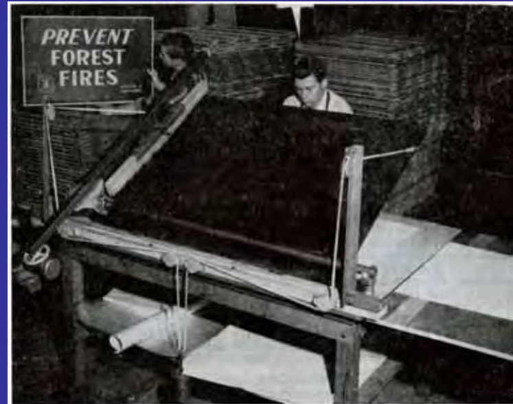
Printing forest fire signs with silk screen equipment.
