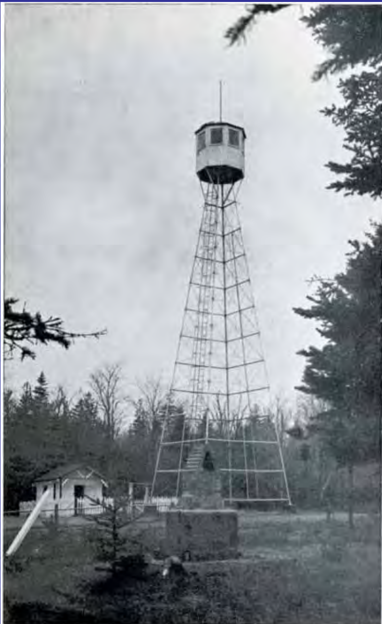
Sixty foot fire tower at Blue Mountain, Pictou County, with adjoining grounds cleared for picnic area. Fire place avoids danger of picnic fires.
